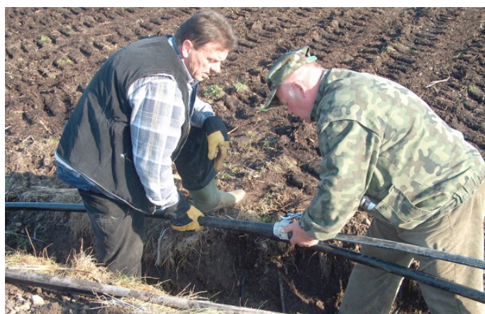
4. Connecting water-pipes
