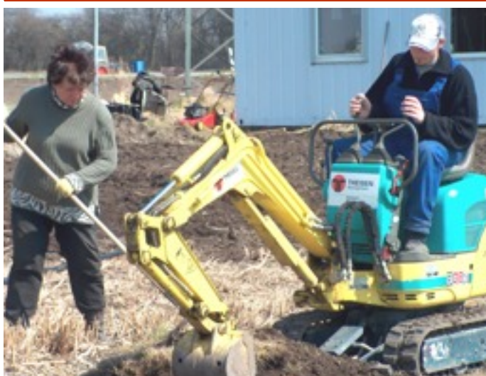
2. Digging trench for water-pipe
